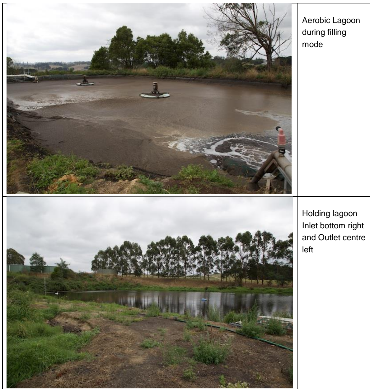
Figure 5-4 Photographs of Aerobic Lagoon and Holding Lagoon
